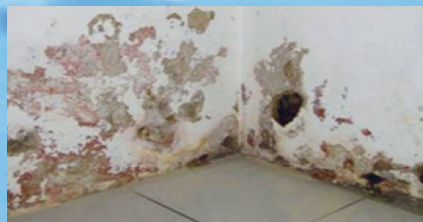
... damage quickly becomes visible in the form of greying and mould formation, etc. ...
